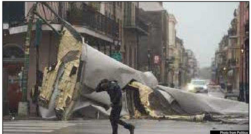
Hurricane Ida wipes out power in city of New Orleans, Louisiana.
