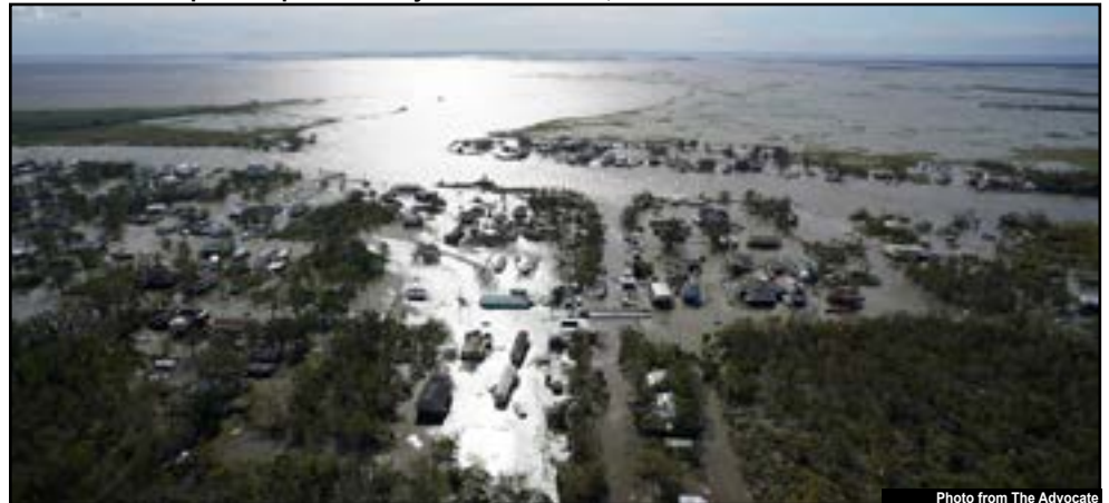
Water damage shown in Lafayette, Louisiana.
