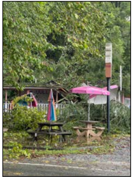
Dolly's Ice Cream Shop building at the entrance to Pisgah National Forest was demolished by fallen trees. (Photo by Olivia Hyde)
