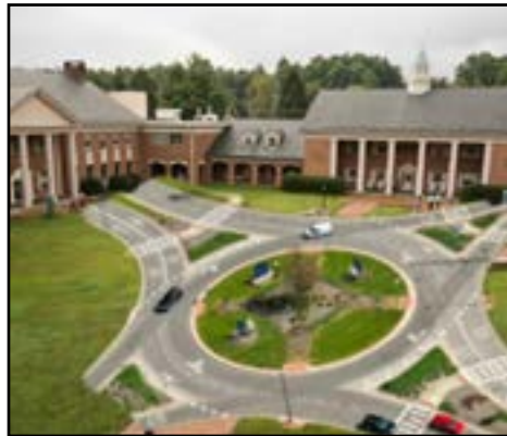
The roundabout in front of Beam Admin.
