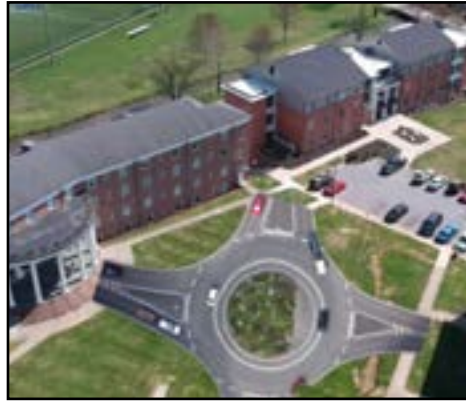
The roundabout replacing one of the quads.
